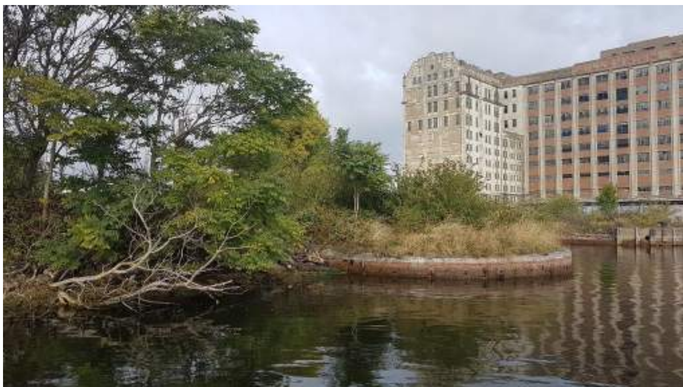
Open Mosaic Habitat of Previously Developed Land habitat around Pontoon Dock and Millennium Mill derelict building ©M Waller
